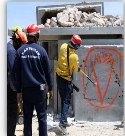
Area 23 Multiple building collapses
